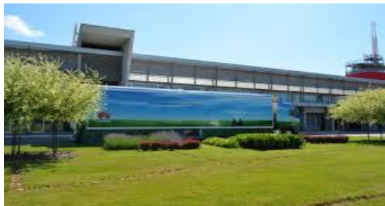
Fig 4: Huawei Cloud Data center.
